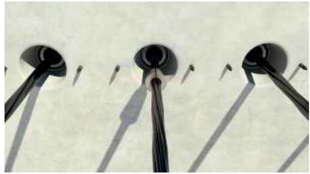
5) Remove former and install block and jaws
