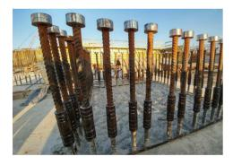
Headcoup Anchorage is designed to create a sufficient hook in concrete based on shear cone theory. It offers an alternative way to create a simpler and more efficient anchorage of the rebar end than the traditional hooked rebar in the concrete. The front face of the coupler is designed to carry the full tension load of the rebar when the anchor is bearing against concrete or structural steel.
