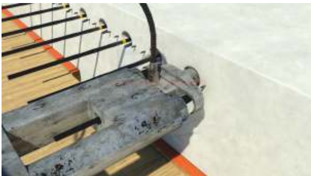
6) Start stressing strands to the value given by the engineer
