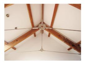
**Regbar Tension Rod** is usually purchased with suitable fork-end dippers for connection to the host structure. Typical applications include hangers and supports, cross linking and shear support elements.
