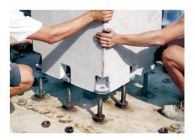
Axis and grade works of foundation manufacturing are completed in the work or project site before the assembly and if there are no problems, assembly process begins. Upon completion of assembly necessary finishes are performed and the building is delivered.
