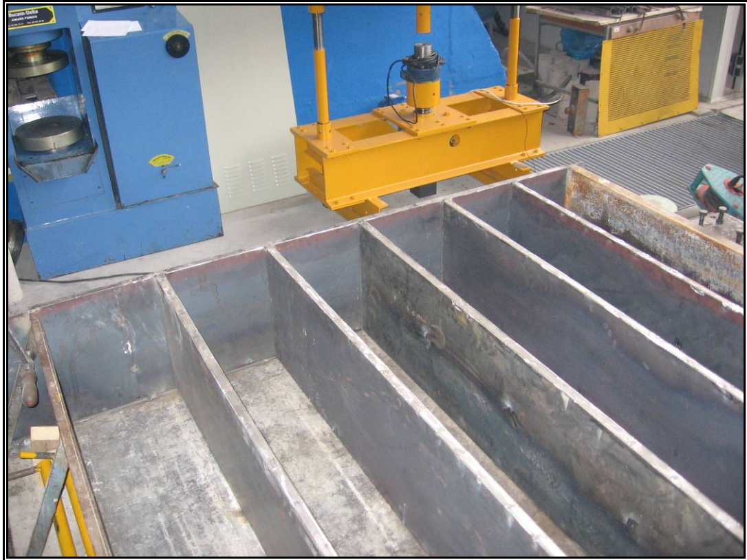
Figure 3.2 Finished view of formwork.
