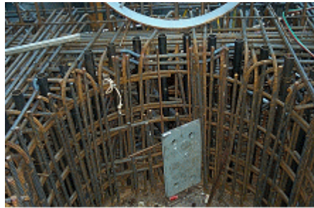
Fig 1. Steel rebar lap joining
