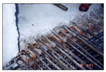
(a) Column bar splicing(b) Splicing of all slab main top barsFig. 6 Typical coupler applications
